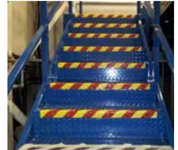
Metal stairs after
